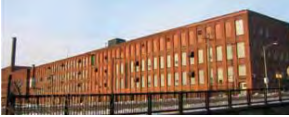
216 Appleton (across the canal). City received $247,000 for cleanup of asbestos and hazardous materials from EPA 9/2013.
